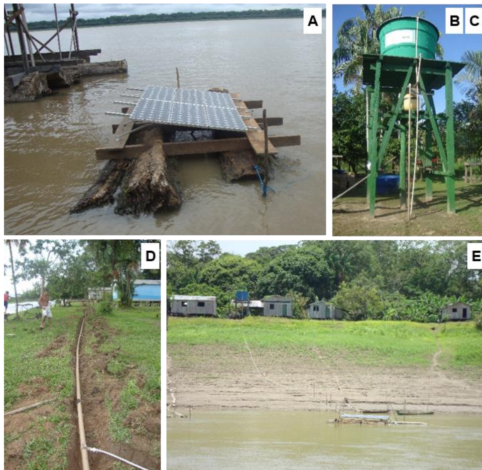
Figure 1. Water supply system operating in RDS Mamiraua
