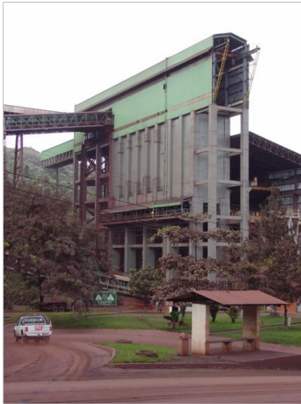
Fig. 2. The Secondary Crushing Facility.
